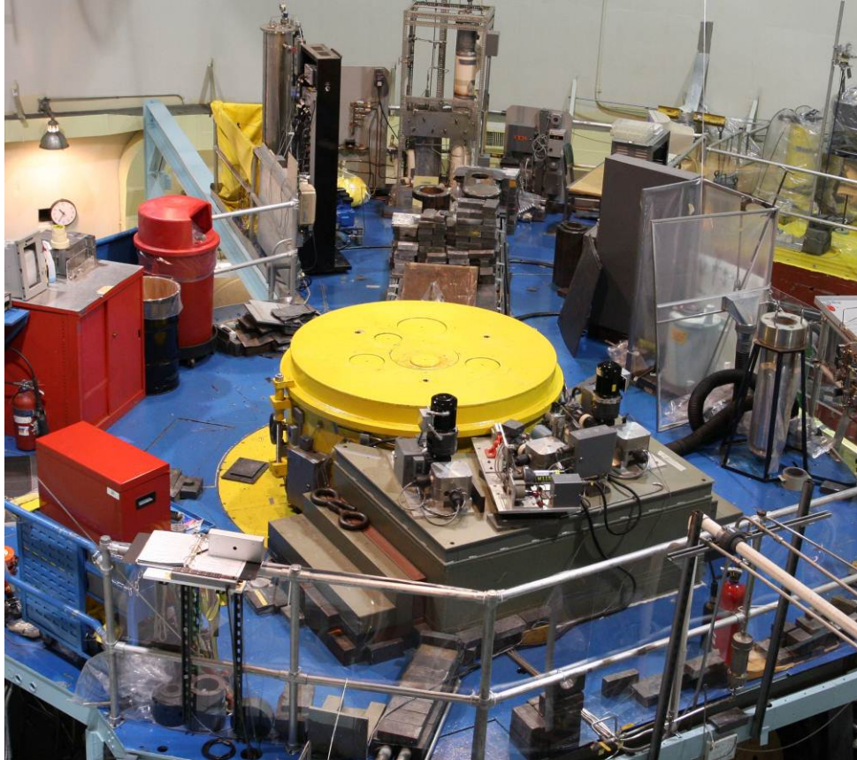
Figure 2. The MITR reactor top.
