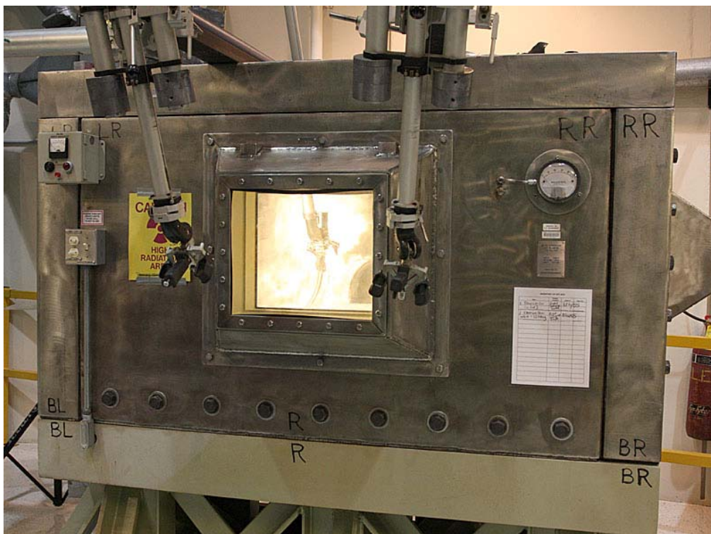
Figure 13. Reactor floor hot box.
