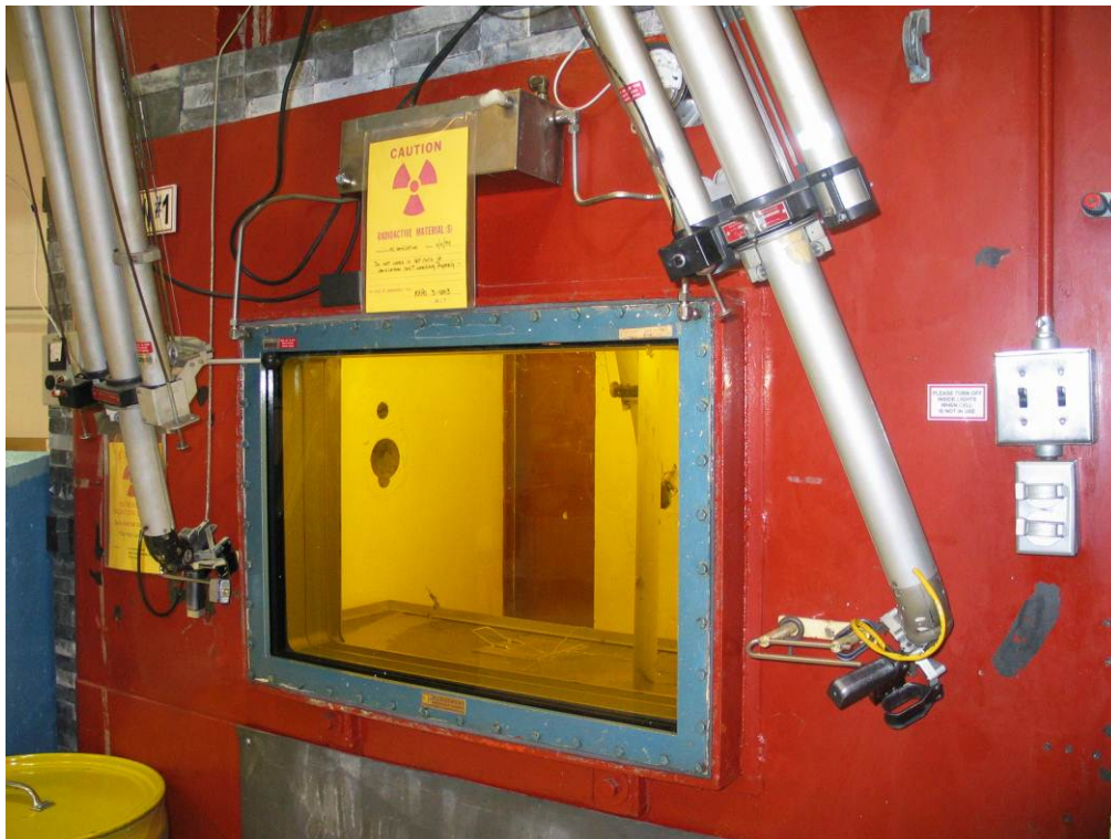
Figure 12. Reactor floor main hot cell.
